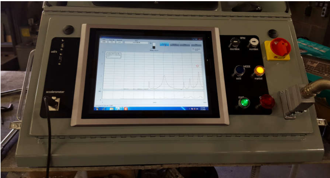
Figure 3: Advanced VSR Model 7.5 Console features a 15" touchscreen PC, 5 HP Allen-Bradley VFD motor drive (with external heat-sink), installed in a NEMA 4 rated enclosure. Flip up / down lid holds a keyboard when open, and covers all controls when closed. Front panel includes a quarter-turn disconnect switch, plus jacks for the accelerometer and vibrator, plus two USB's.
