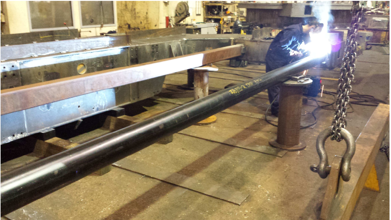
Figure 7: After the two VSR Treatments, which completed the stress relief, braces spanning the space between the structure’s “arms” were cut. Dimensions had been mapped of a triangle spanning the braced area, and these dimensions were taken again after brace removal. Results shown in Fig. 8
